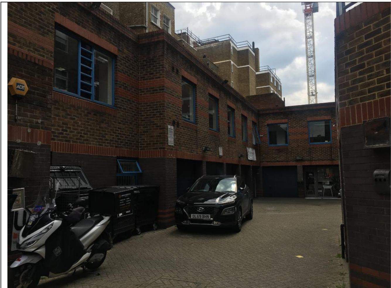
Photograph of existing Olympia Mews to rear of Queensway
