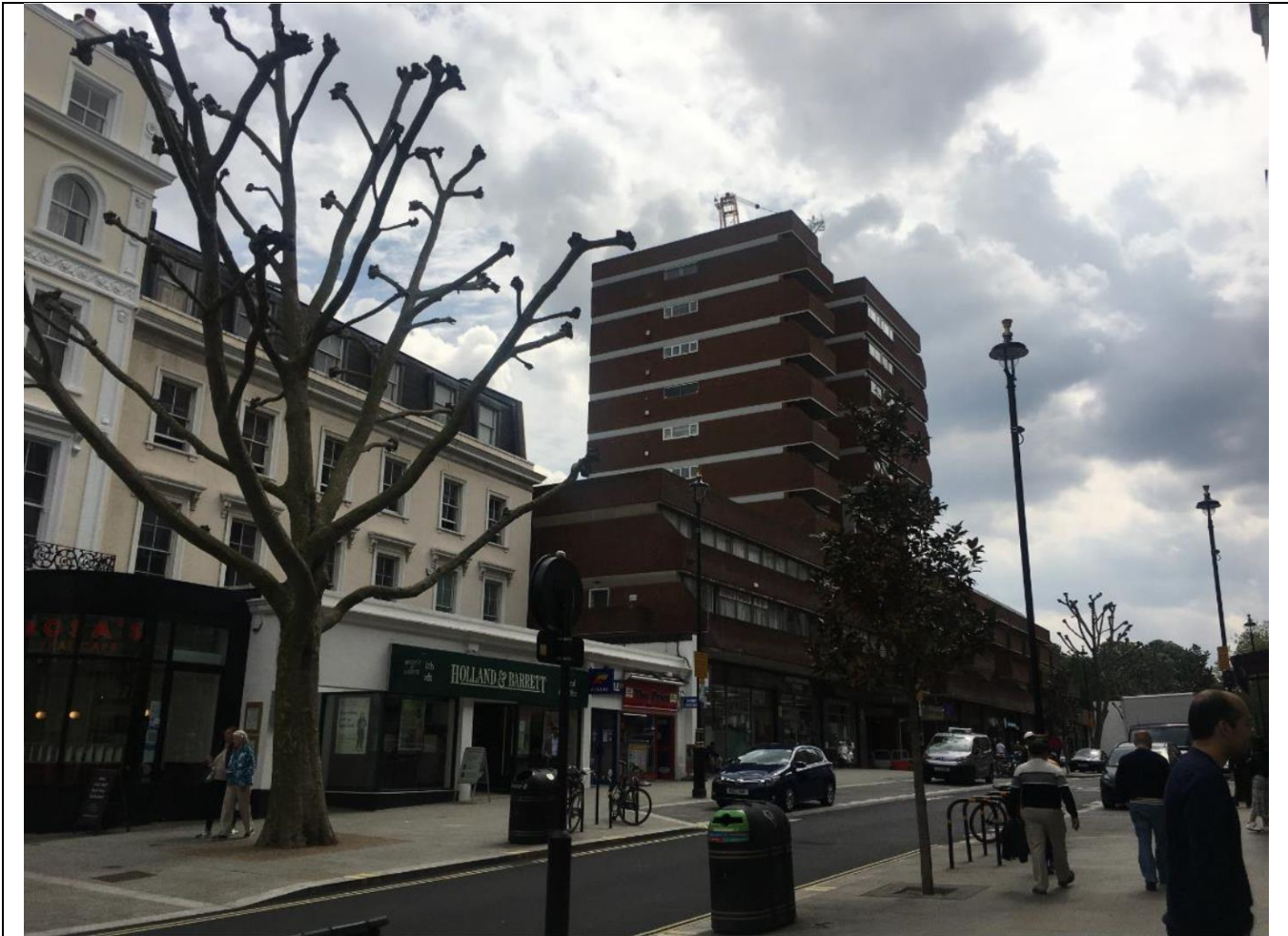
Photograph of existing front elevation to buildings on Queensway
